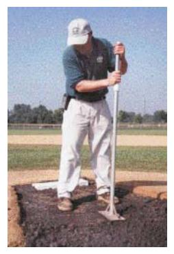
Apply 1" layer of Pro Mound to each area and tamp to compact. Water and allow to soak in before repeating in 1" layers to within 1/2" of finished grade.
