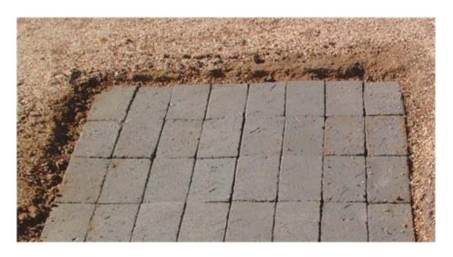
Water the areas and allow to soak into the bricks for 1-2 hours.
