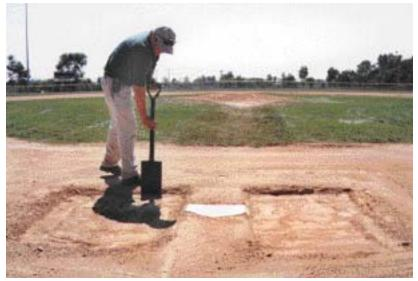
Remove top 4-6" of top soil from area around and in front of rubber in mound.
