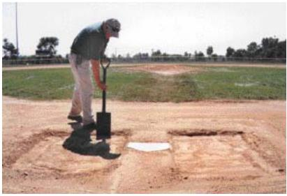
Remove top 3-4" of top soil from area around and in front of rubber in mound.
